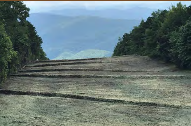
Energy / Pipeline Restoration
