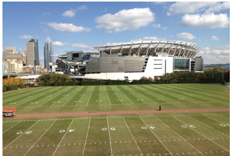
Photos: Surface being prepared and graded; Completed fields after construction and grow-in.
